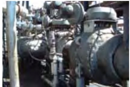
This midwestern refinery has four 20-inch ASME 300 class MOGAS ball valves in overhead vapor service. Several are beginning their second decade of service.
