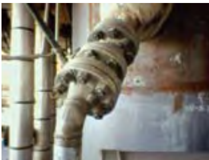
This CA-DRI 2-inch ASME 300 class isolation valve handles the withdrawal of hot spent catalyst from the regenerator.
