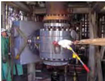
This 16-inch 600 ASME class valve was installed for 550° F at 1095 psig (290° C at 75 bar g) lockhopper isolation service. Several of these valves withstood over 50,000 cycles.
