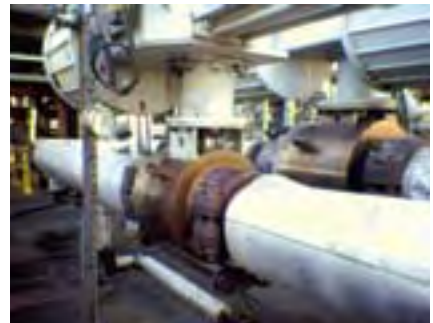
These 12-inch and 16-inch ASME 2500 class floating ball valves are installed at the letdown station of a European refinery responsible for producing 115,000 bpd.
